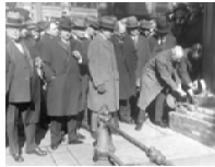
Tearing down the Ebbitt Hotel to make room for the National Press Building Jan. 6, 1926
