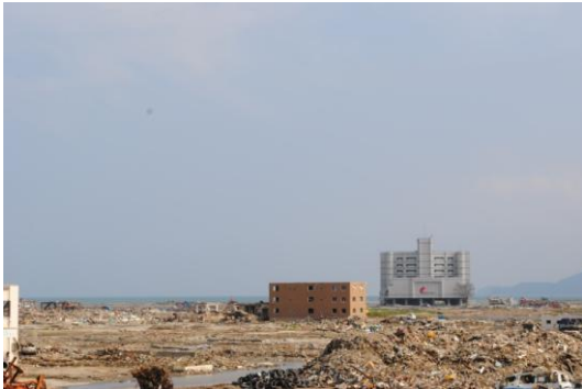
The Capital Hotel (Sen Masao) stands in the ruins near the sea. Taken from the tsunami-hit city hall building.
