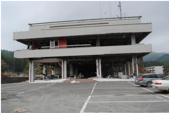
The tsunami-ravaged Onagawa Town Hall building (Taken on June 2, 2011).
