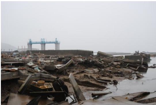
A seawall and floodgate near Shizugawa Port (Taken on June 2, 2011).
