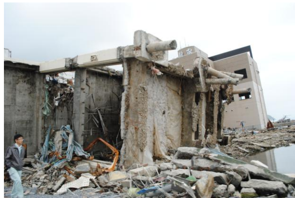
This building toppled over along with its foundation (downtown Onagawa).
